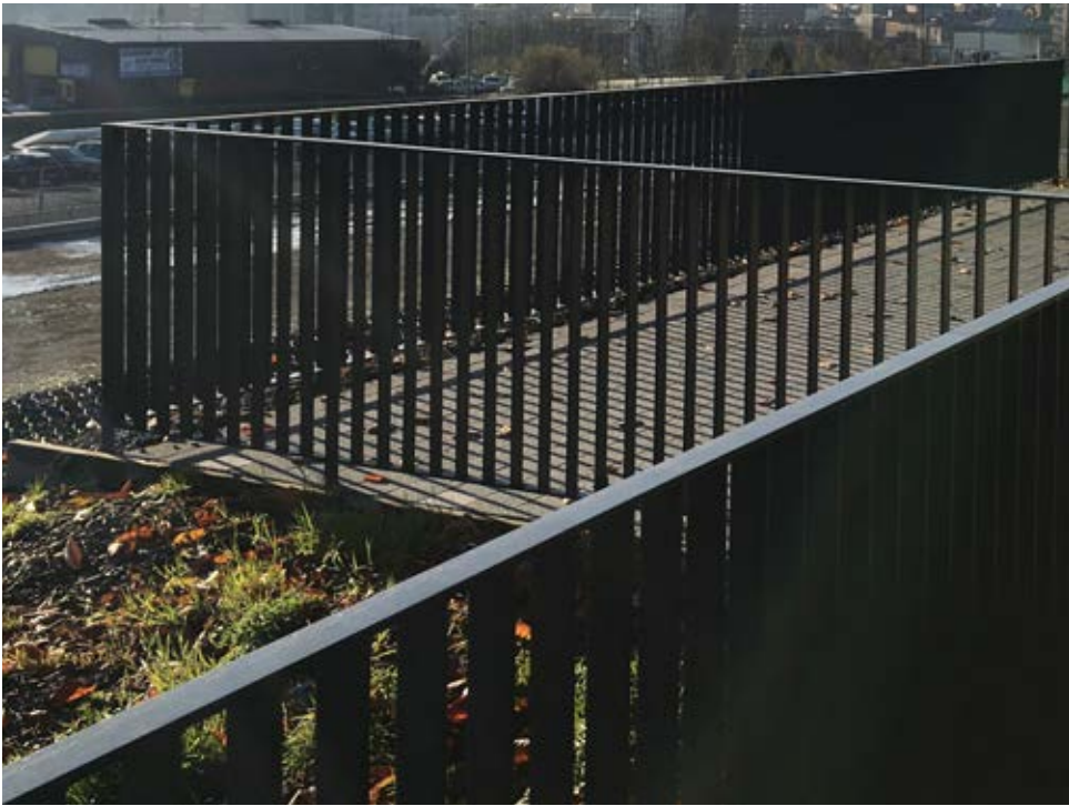
Fall protection barriers using open steel railings rather than brick parapets increase visibility and give a sense of openness
