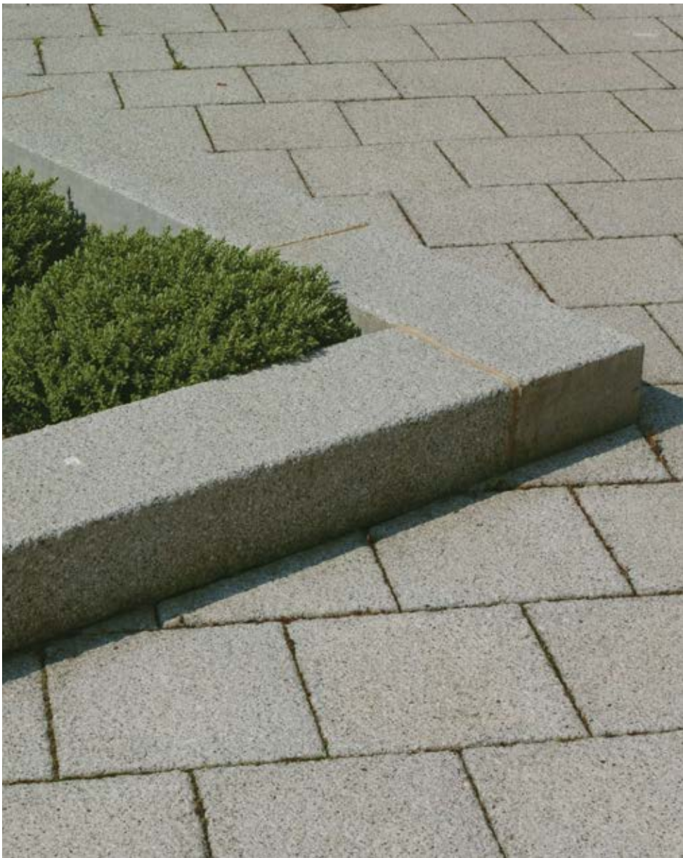
Marshalls Conservation kerbs will form the upstand to the space.
